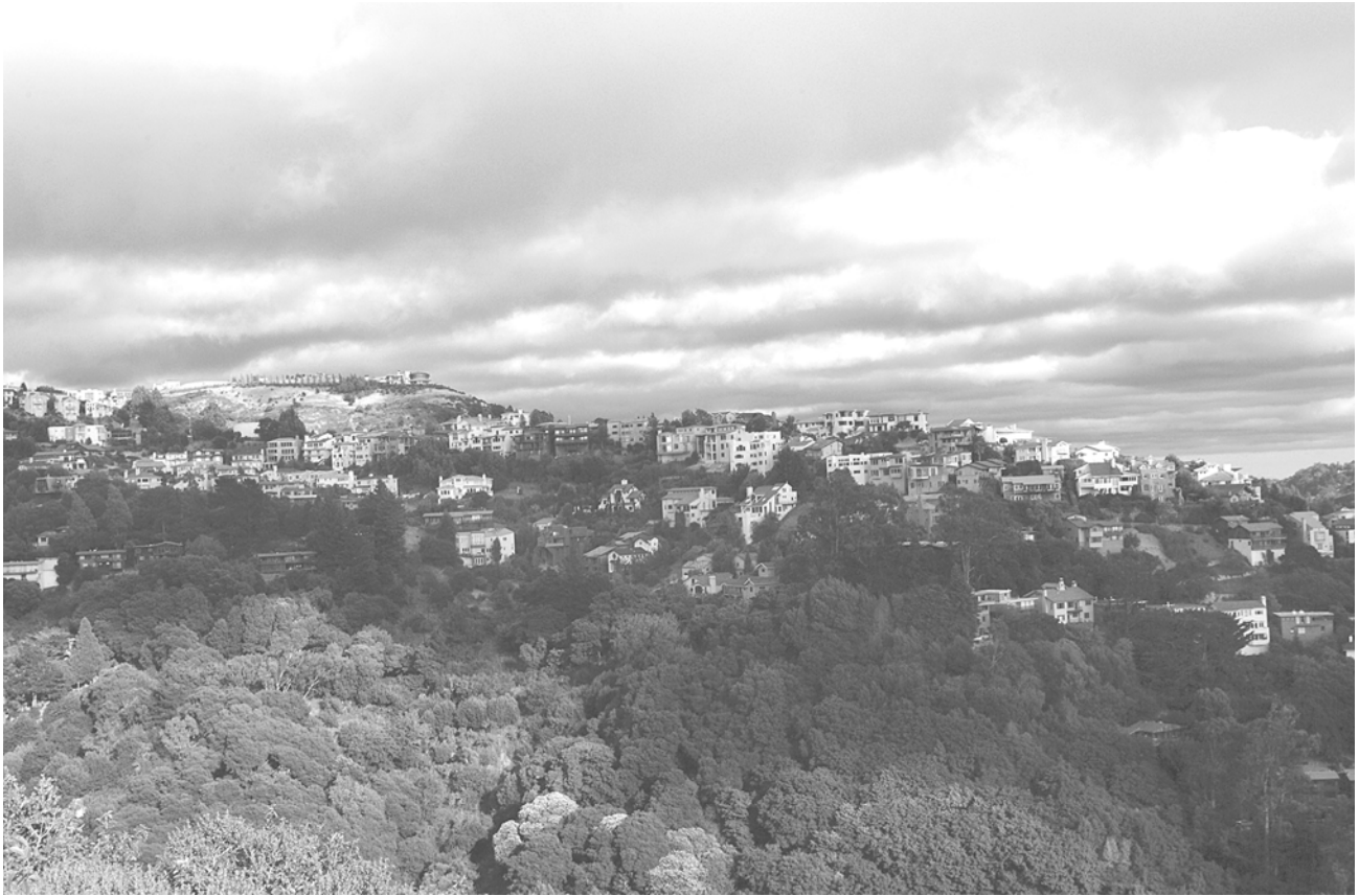
Homes at the urban-wildland intermix, as seen from the Ridge Trail of the Claremont Canyon Preserve, stand out against the cloudy sky. Just below the homes, most of which were rebuilt after the 1991 firestorm, is the mixed hardwood forest of Garber Park. The entirety of Garber Park was spared during the firestorm.
