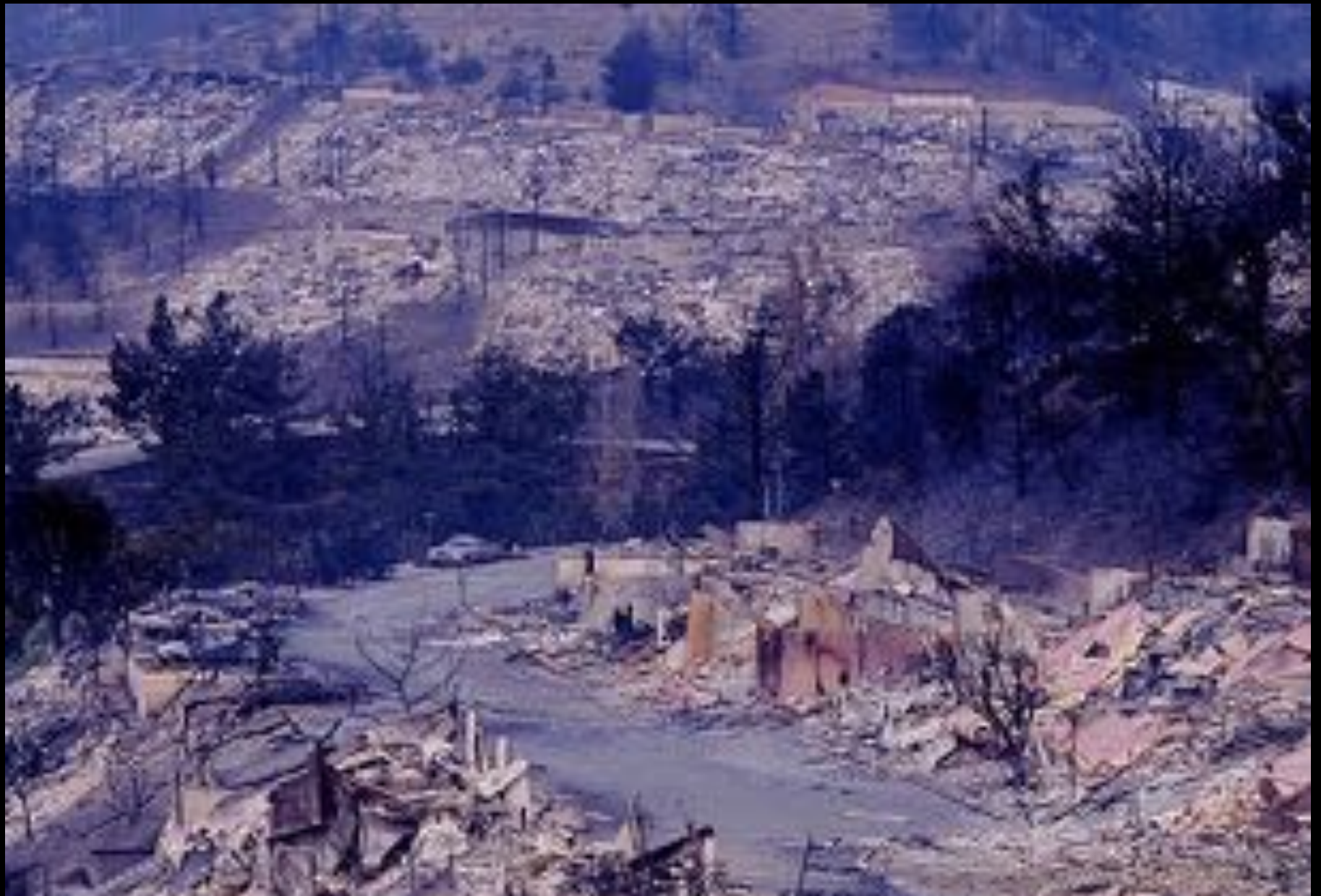
HILLER HIGHLANDS AFTER THE 1991 FIRE
