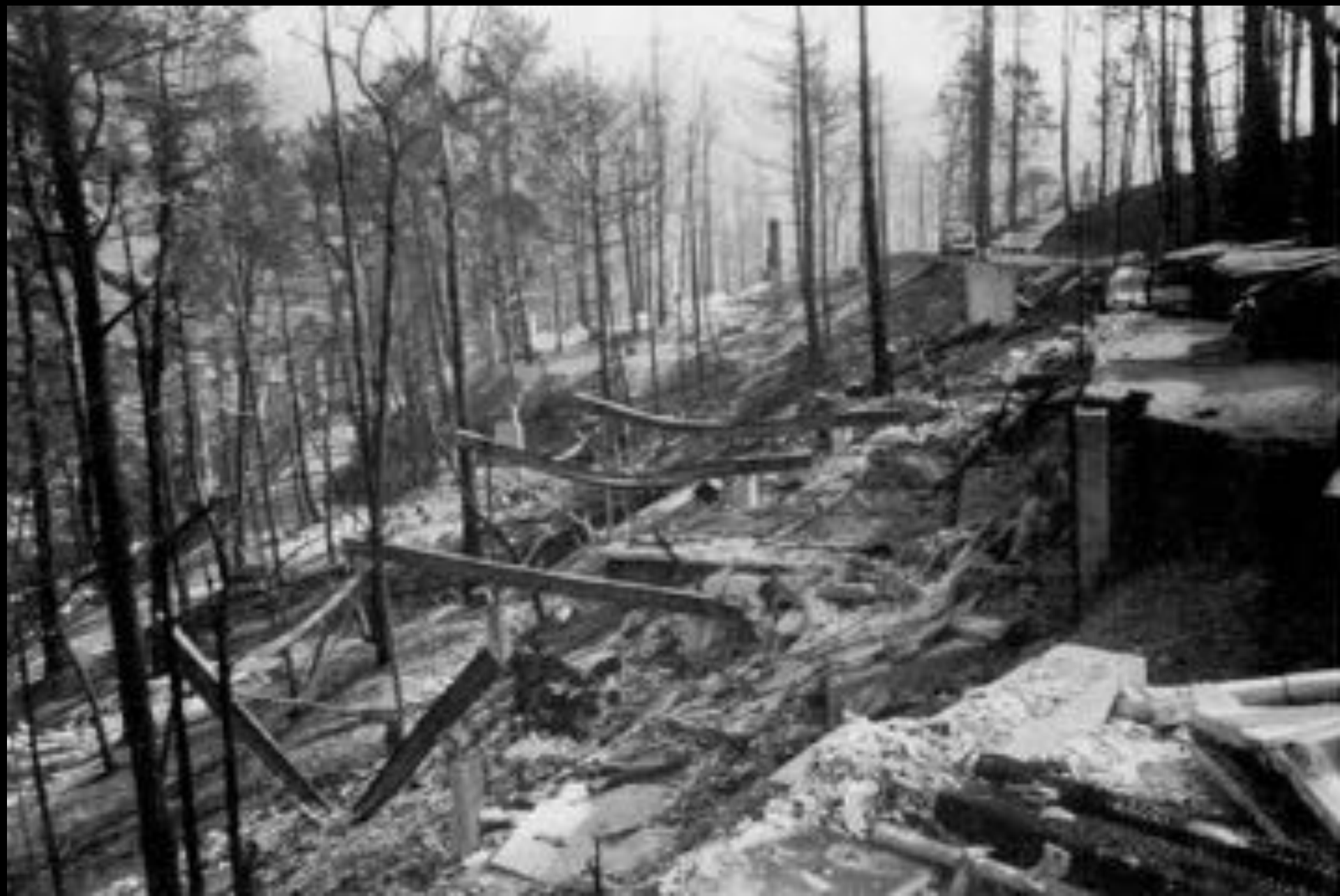
DESTROYED RESIDENCE SURROUNDED BY PINE TREES ON BUCKINGHAM AFTER THE 1991 FIRE
