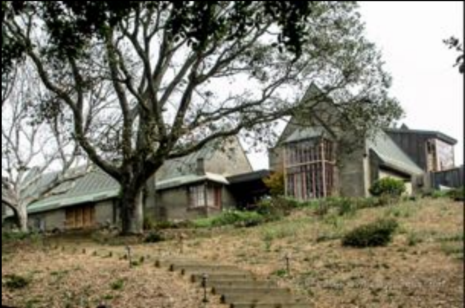
Maybeck's 1937 Wallen- His son's home above Wildcat Canyon GOAL: RAIN AND FIRE PROOF WITH METAL ROOF AND CONCRETE SIDEWALLS Note: oak trees with great defensible space in 2016
