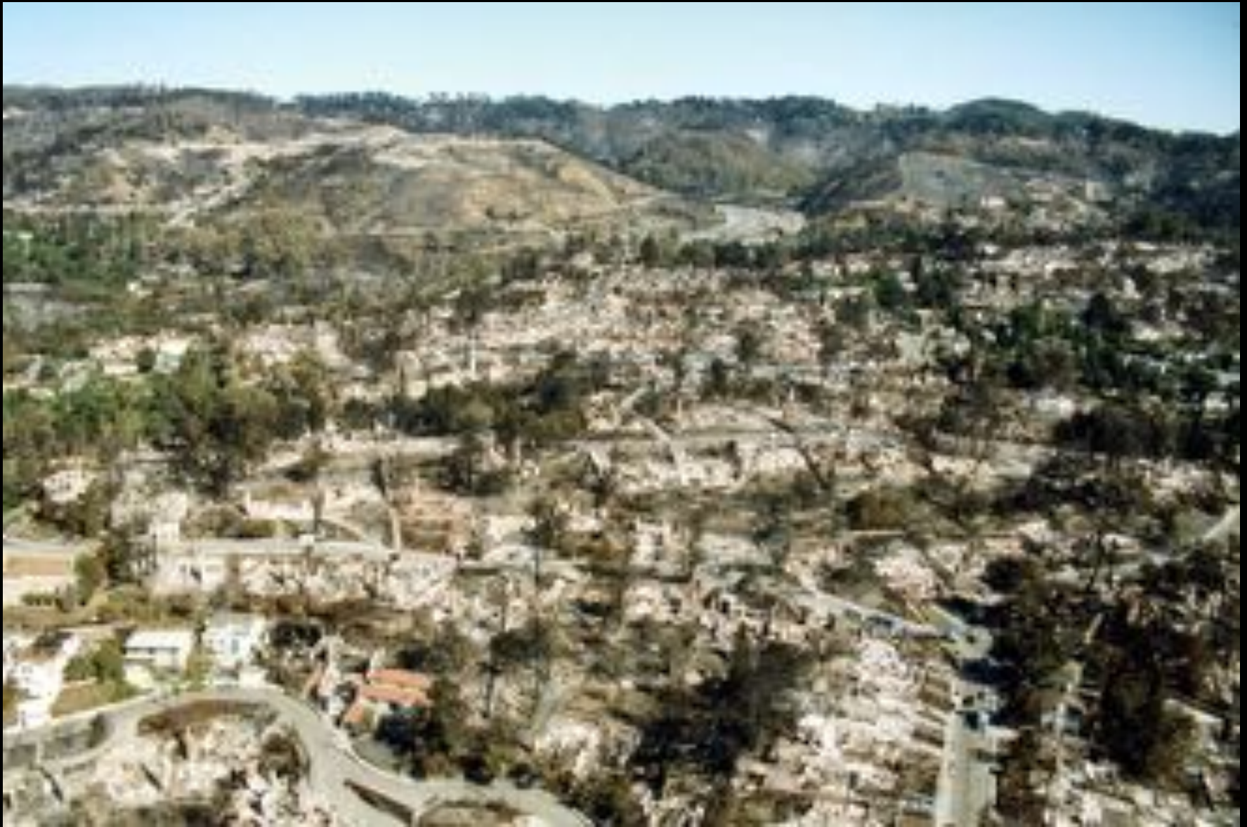
UPPER ROCKRIDGE AFTER THE 1991 FIRE
