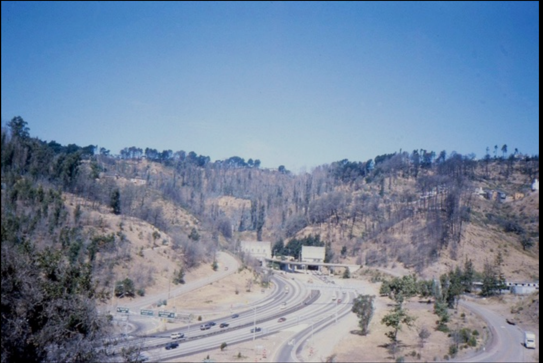
TUNNEL CANYON AFTER THE 1991 FIRE
