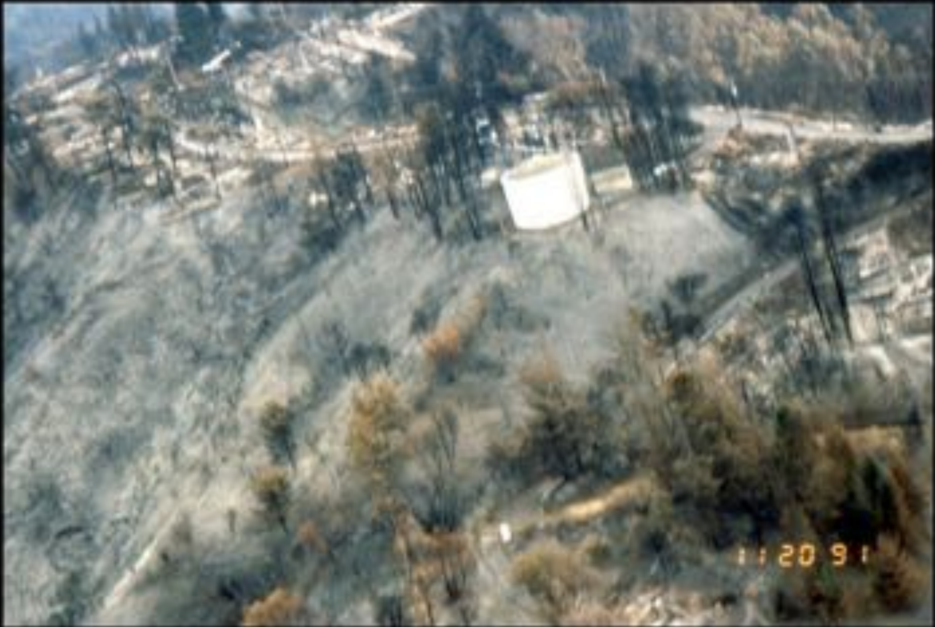
THESE HOMES DID NOT SURVIVE THE FIRE IN GWIN CANYON
